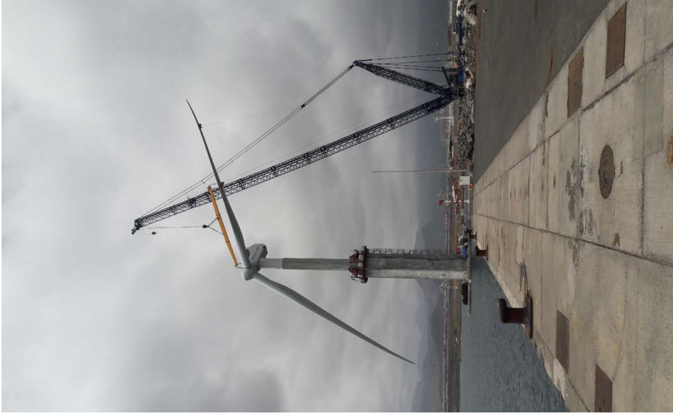
WTG Installation onto a Gravity Foundation in Port
